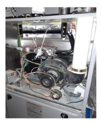
COMBINATION SYSTEM: provides basement floor heating via hot water radiant
