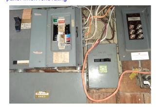
BRANCH WIRING: some areas with ungrounded wiring though no knob and tube observed during random sampling, upgrade when renovating
